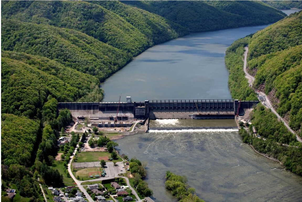
Figure 1. General view of dam with 6 penstocks (left hand side) with thrust blocks and stop logs being installed. (courtesy: Public Affairs, USACE, Huntington District).
