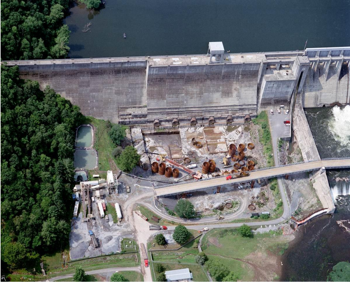
Figure 5. Photo showing the penstock area in detail, before installing the thrust blocks. (courtesy: Public Affairs, USACE, Huntington District).
